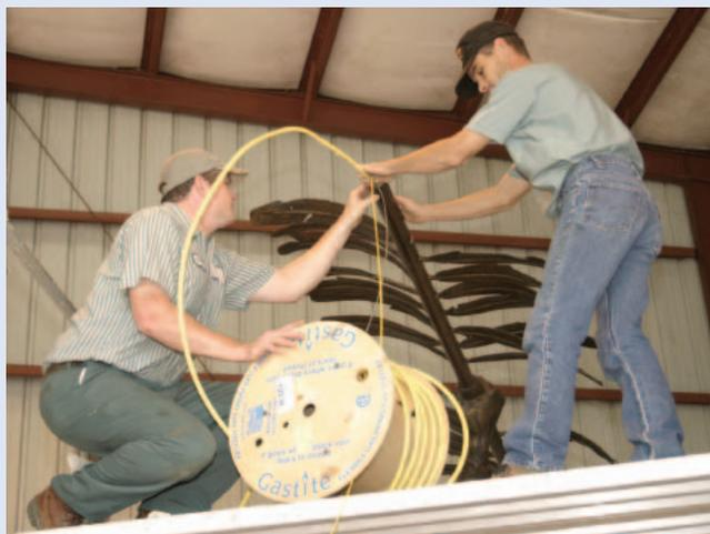
Installers thread Gastite flexible gas piping into the spear of "Unconquered."
